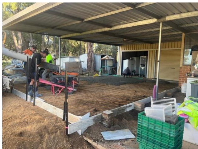
Preparation and pouring of slab for cool room
